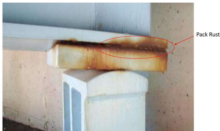
Figure 2.13. Pack rust on a rocker bearing
